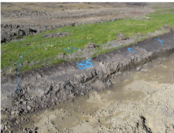
Figure 6 By continuous checking edges and base of the excavated hotspots certainty is gained about the remaining soil which will be brought to the mixing pile.
